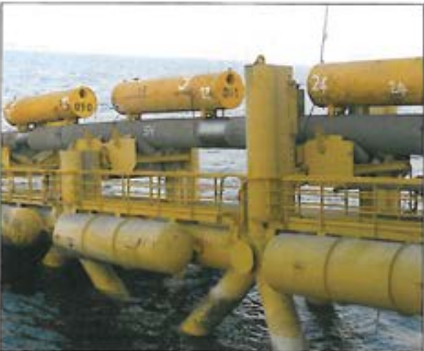
A view of the pipeline along with Buoyancy Tanks aboard The Singer
