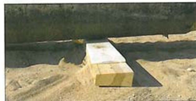
General view of a wooden traverse with a polyamide sheet
