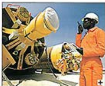
Workers inspect some of the massive suction piles that help stabilize the FPSO.
