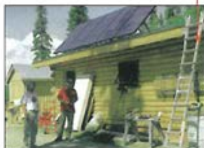
During non-winter months, solar photovoltaic arrays provide clean, quiet electricity for bunkhouses, storage sheds, and other buildings at BLM's remote Chicken, Alaska, Field Station.
